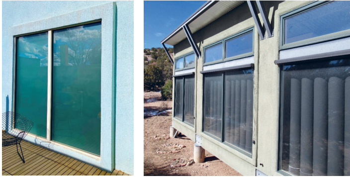
Figures 26–27. One of two Trombe walls in Davis House 3 (figure 26, left) and the Sol-Mod's Trombe wall seen from the outside, composed of an array of vertical PVC tubes filled with water, painted black on the outside and white on the inside (figure 27, right). (Photographs by Bruce Davis, circa 2010.)
