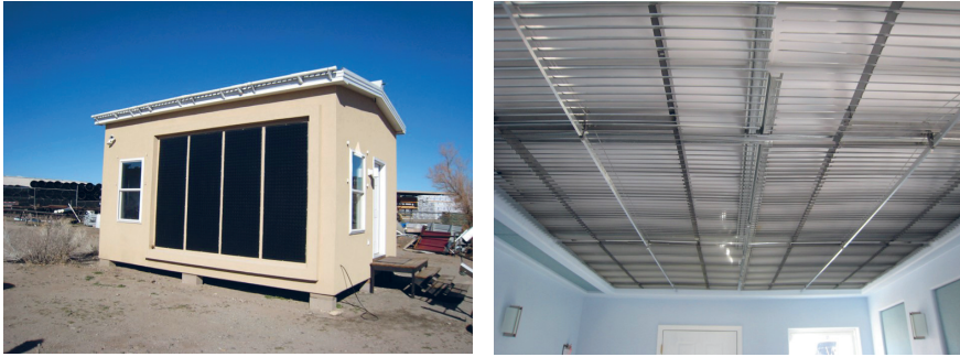
Figure 24–25. The Dave House, built on Zomeworks grounds circa 2007, with 4 solar collectors on the façade and a more cleanly integrated rooftop radiator when compared to the Andy Shack (figure 24, left), and the sub-ceiling PVC array in the Dave House, with aluminium louvers below, replicating the same array seen in the Andy Shack, and marking Baer’s abandonment of the vertical water array (figure 25, right). 71
