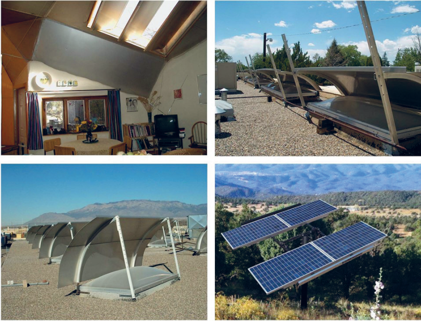
Figures 2–5. The Skylid insulated louver system installed in the Baer residence circa 1973 22 (top left, figure 2); the Sunbender reflector/shading system installed in Bruce Davis House 2, in the summer position, circa 1990s 23 (top right, figure 3); the same Sunbender system at the Zomeworks Corporation headquarters, in the winter position, circa 1988 24 (bottom left, figure 4); and the UTRF-072 model of the TrackRack passive photovoltaic tracking system, date unknown 25 (bottom right, figure 5). (Photographs by Zomeworks Corporation.)
