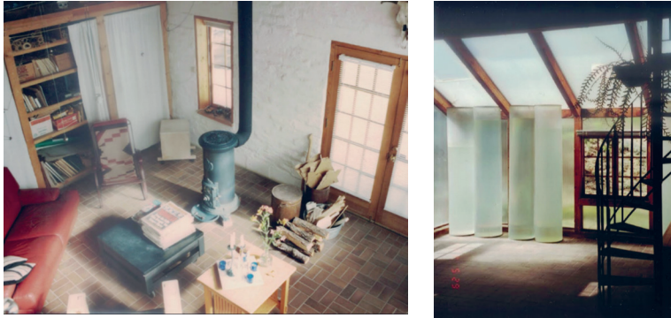
Figures 12–13. Interior view of the eastern wall of the residence (figure 12, left), and interior view of the water cylinders facing the south-facing fenestration (figure 13, right). (Photographs by Bruce Davis, circa 1980s.)
