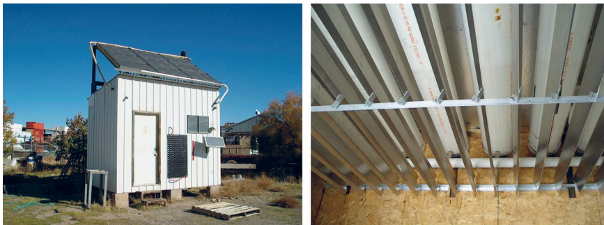
Figures 16–17. Exterior image of Andy Shack, constructed 1988, with the rooftop radiator composed of pig mats visible (figure 16, left), and interior image depicting the sub-ceiling interconnected 8" PVC array, and the aluminium louvers in their open position below (figure 17, right). 54
