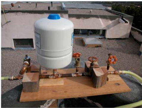
valves, expansion tank, and pressure relief
