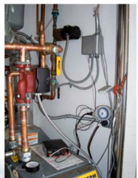
view of mechanical closet
