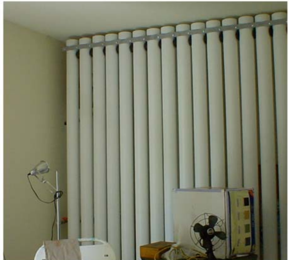
Interior PVC thermal radiators be large in diameter to allow for thermosyphoning
